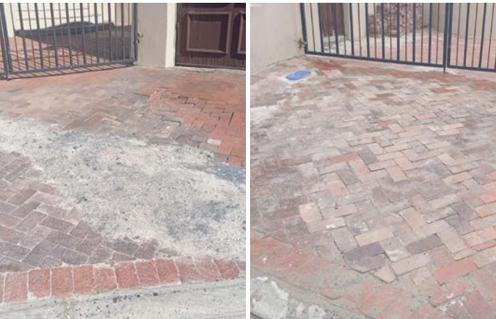
Hole's whole again: Before-and-after shots of a paving reinstatement. The City has been hard at work across town fixing paved surfaces where emergency digging had to be performed.
